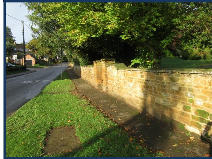
Figure 38: Stone boundary wall to Home Farm, Brixworth Road
