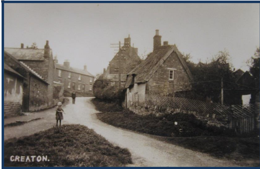
Figure 14: The High Street looking SW from the junction with Brixworth Road
