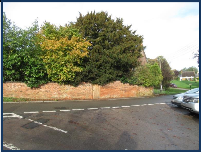
Figure 36: The brick boundary wall at The Manor House
