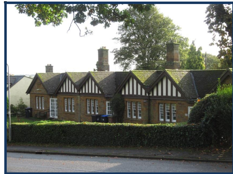
Figure 35: Part of the hedgerow boundary on the southeast side of The Green in front of the Almshouses
