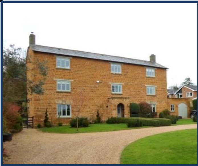
Figure 58: Court House, 4 Court House Close
