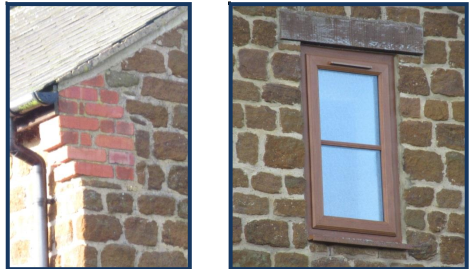
Figure 48: Brick kneeler (left) and timber lintel above window (right)
