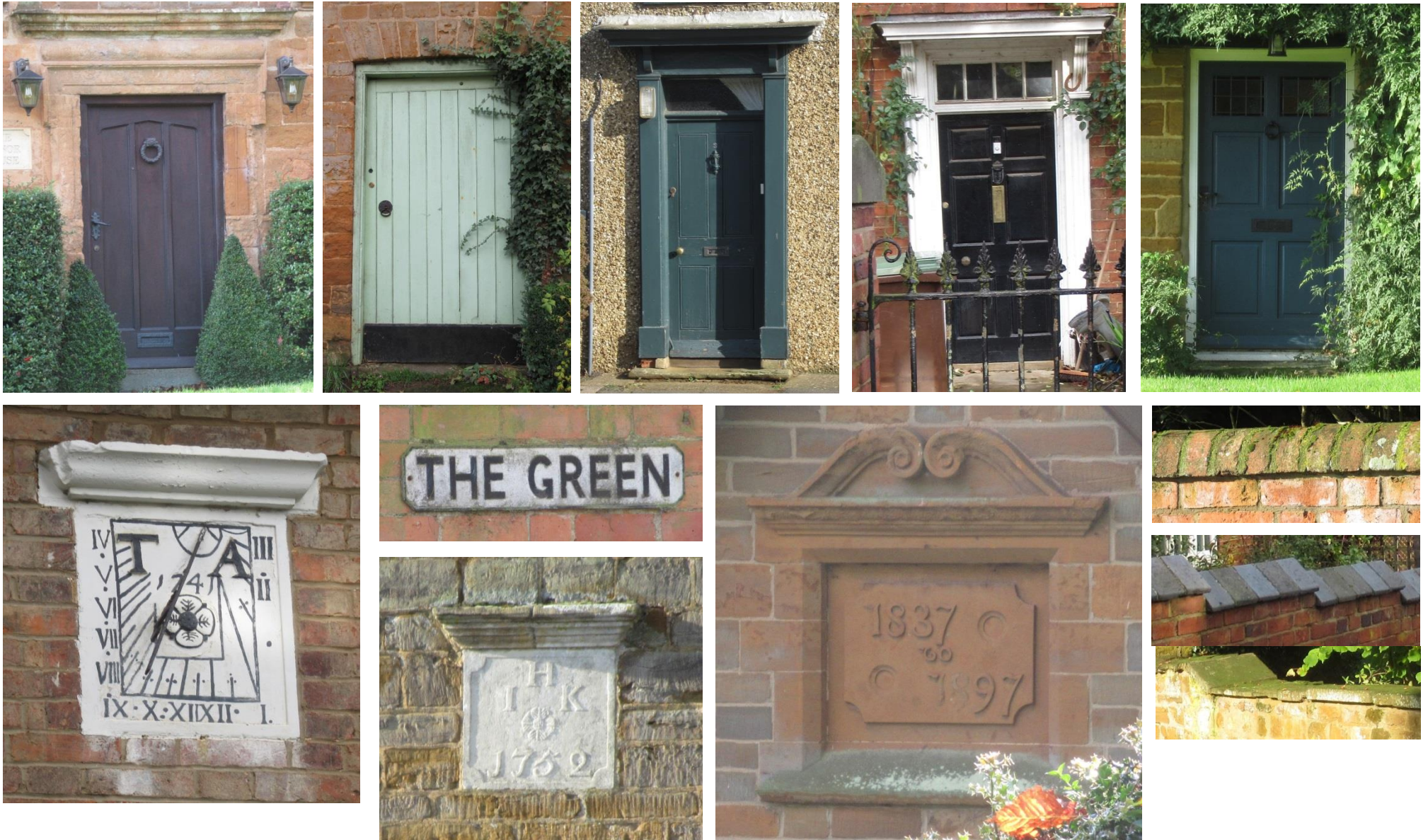
Figure 41: A selection of images showing typical materials, surfaces, boundary treatments and fixtures which form a representative palette for Creaton Conservation Area.
