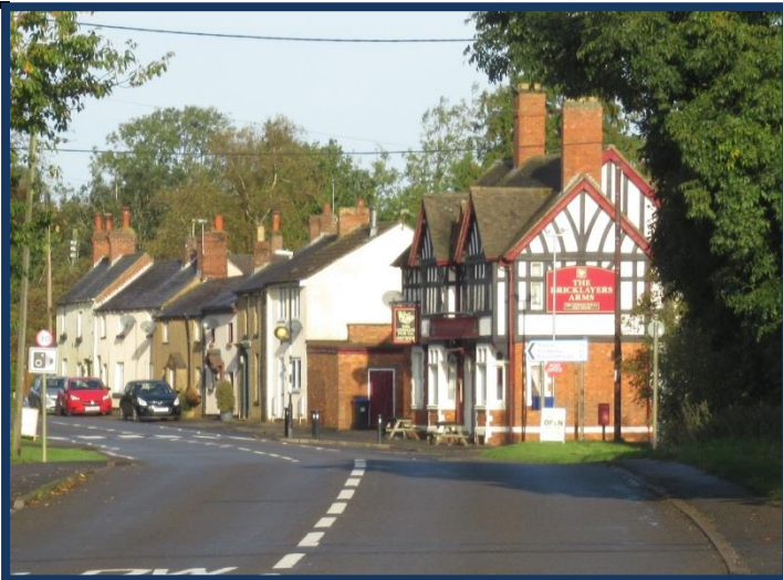
Figure 44: Slate roofs and varying ridge lines of cottages on Welford Road
