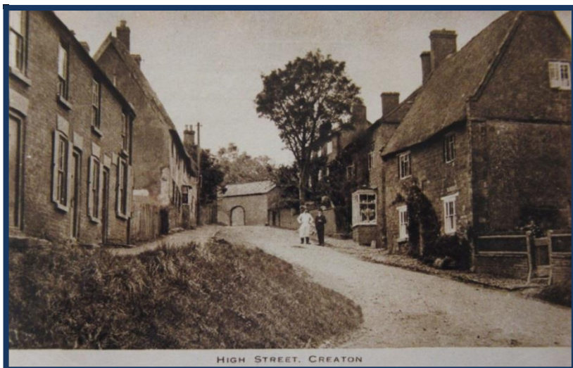
Figure 10: The High Street looking southwest from the junction with Horseshoe Close, 1920
