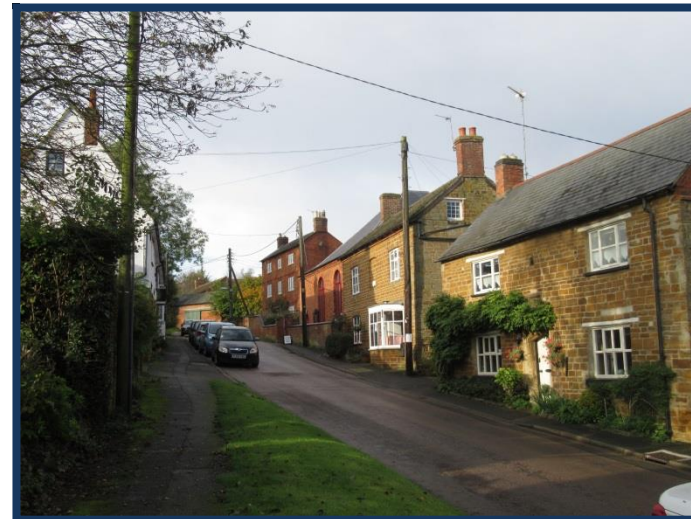
Figure 64: Telegraph poles and overhead lines, High Street
