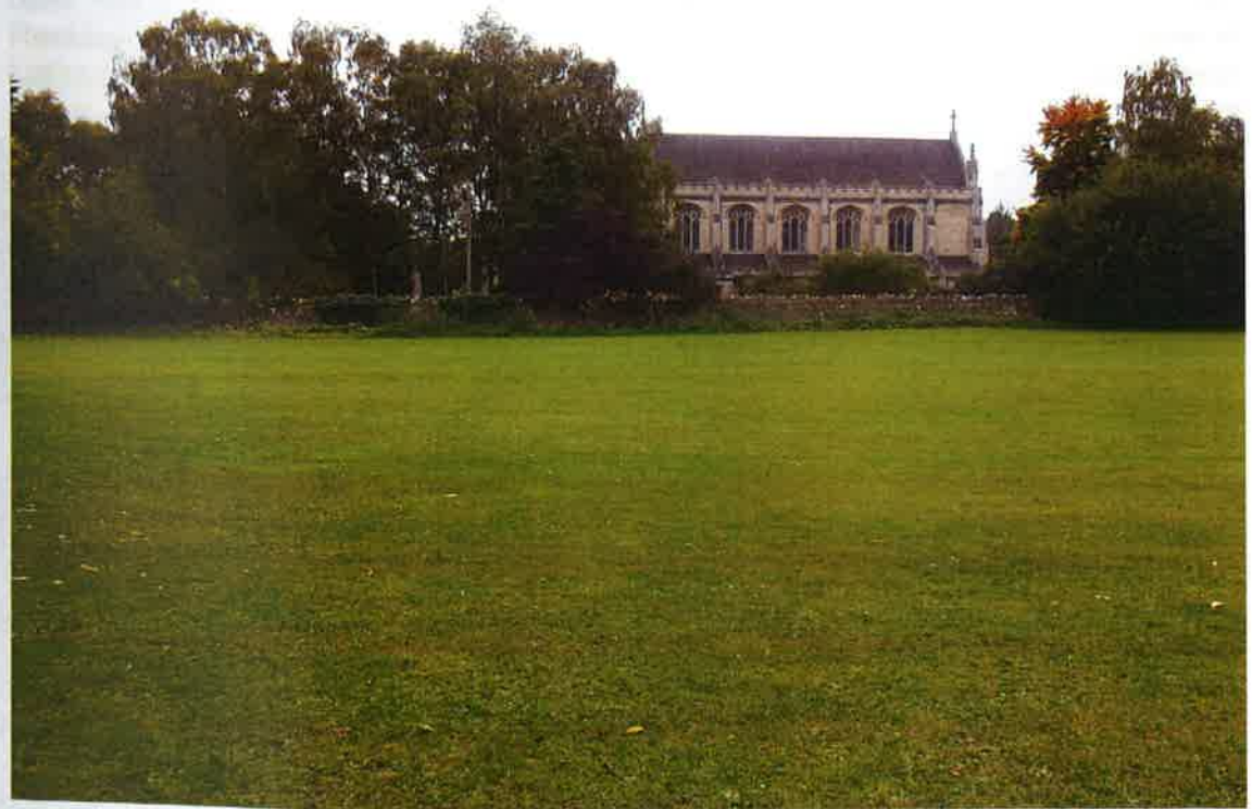
View of southern boundary and Oundle School Chapel, looking south Fig 4
