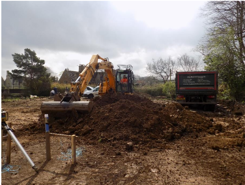
Figure 3: Site monitoring, looking south
