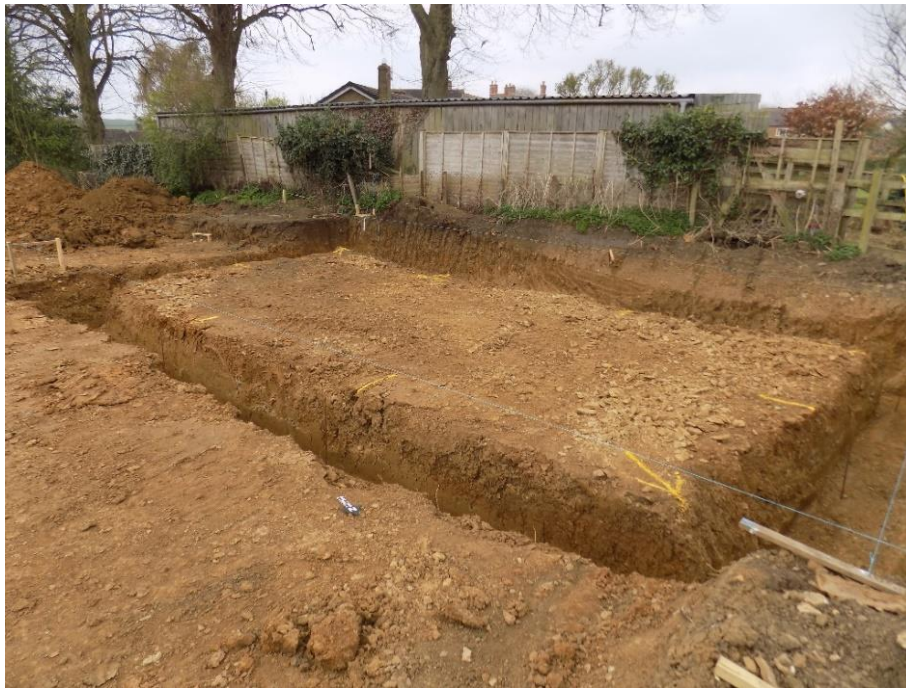
Figure 10: Finished foundations of the garage area, looking southwest
