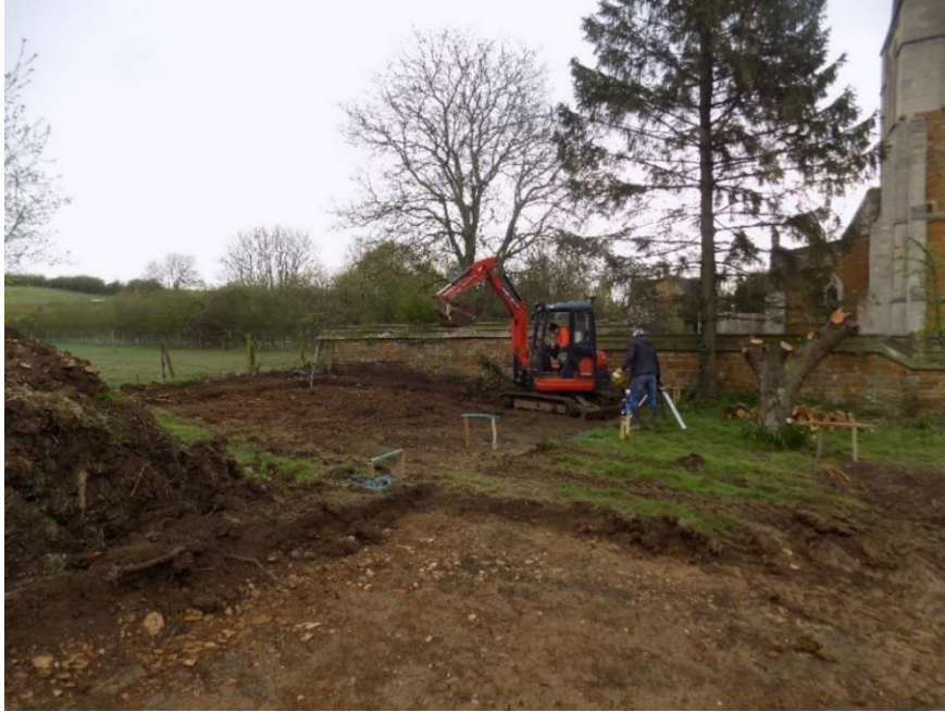
Figure 8: Machine excavating the north-south trench of garden store, looking north-east
