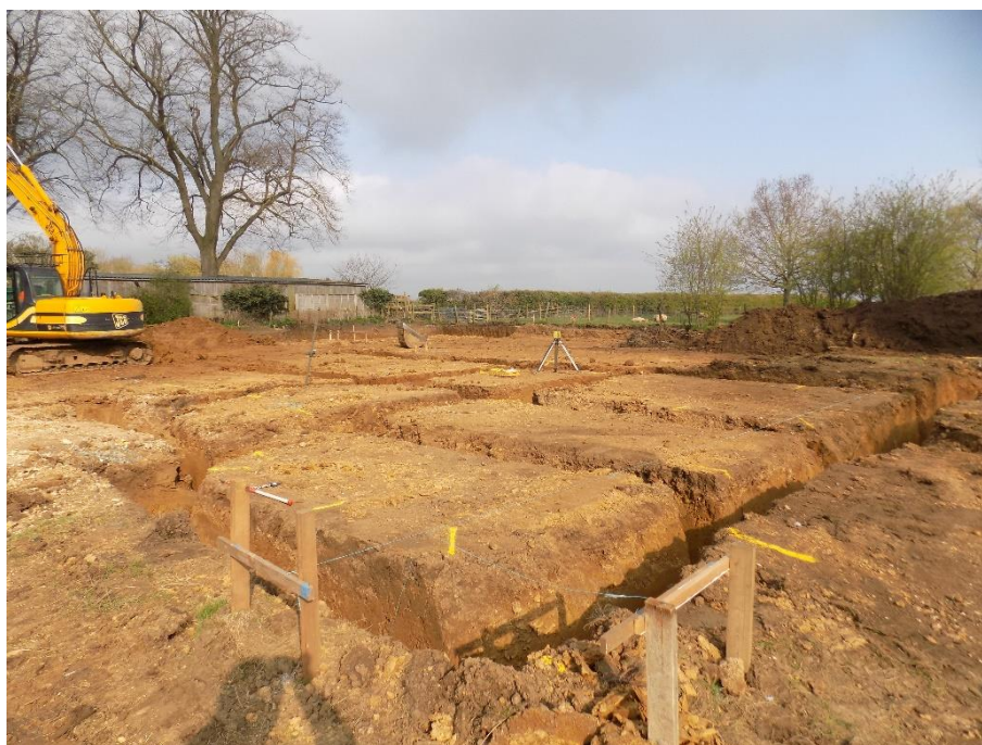
Figure 13: Finished foundations of the house, looking northwest.
