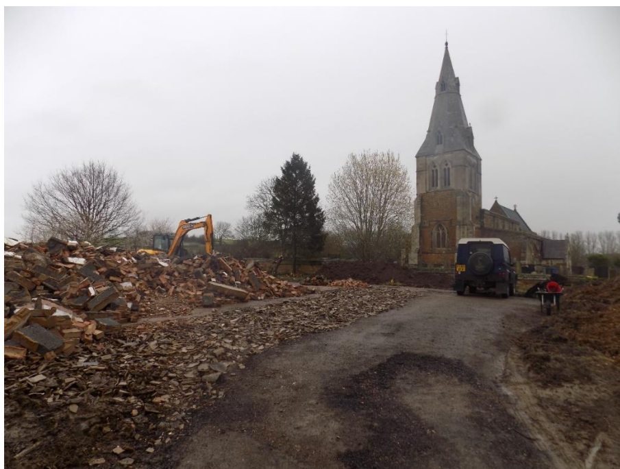
Figure 6: Aftermath of the demolished bungalow and garden, looking north-east
