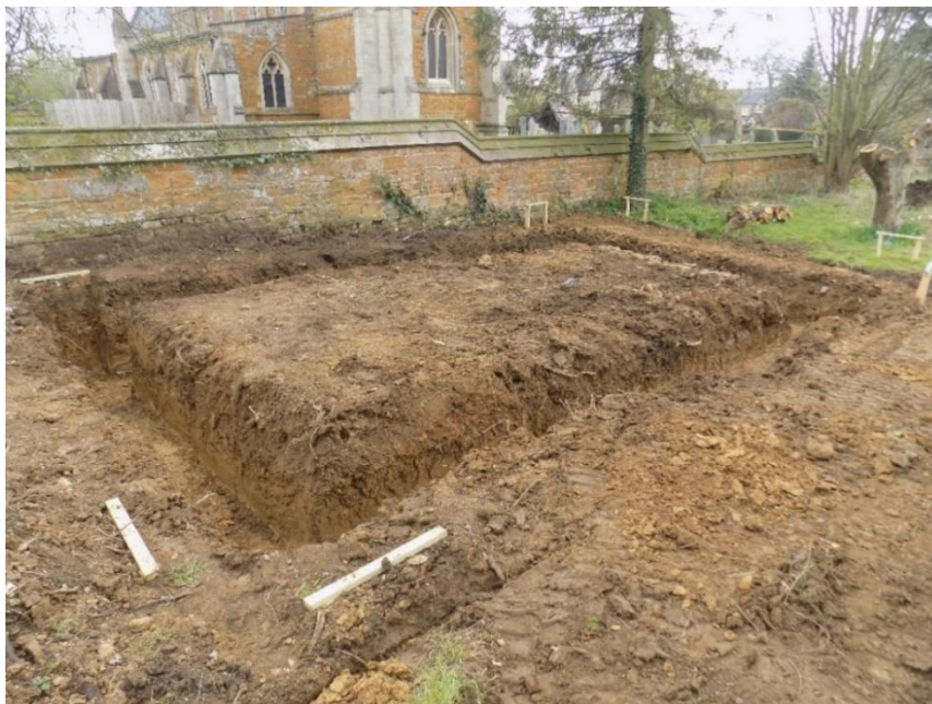
Figure 9: Finished foundations of the garden store, looking south-east
