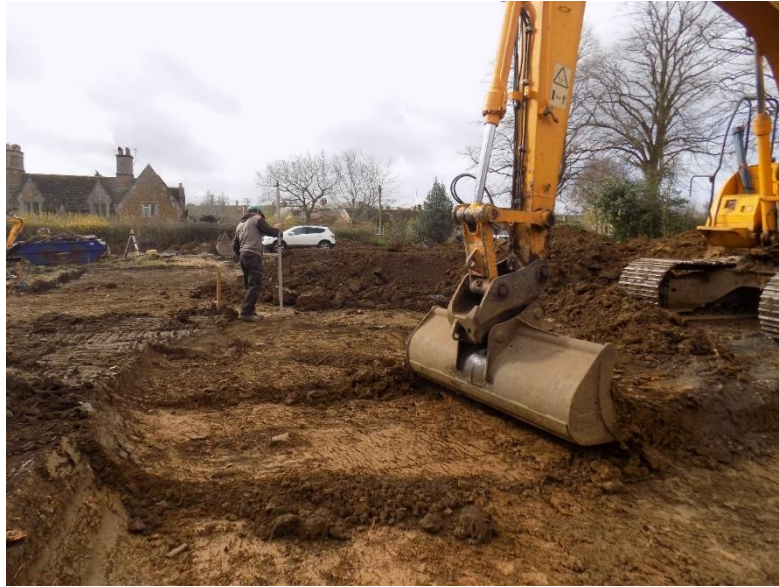
Figure 5: Stripping the northern to central area of the site, looking south
