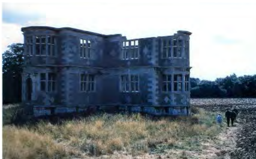
Fig. 5/30 The New Bield with ploughing close to the structure, 1960s
