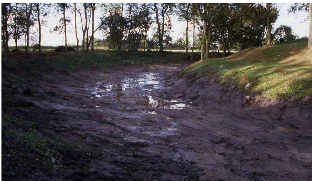
Fig. 5/32 Photograph of moat profile taken in the 2000 de-silting works
