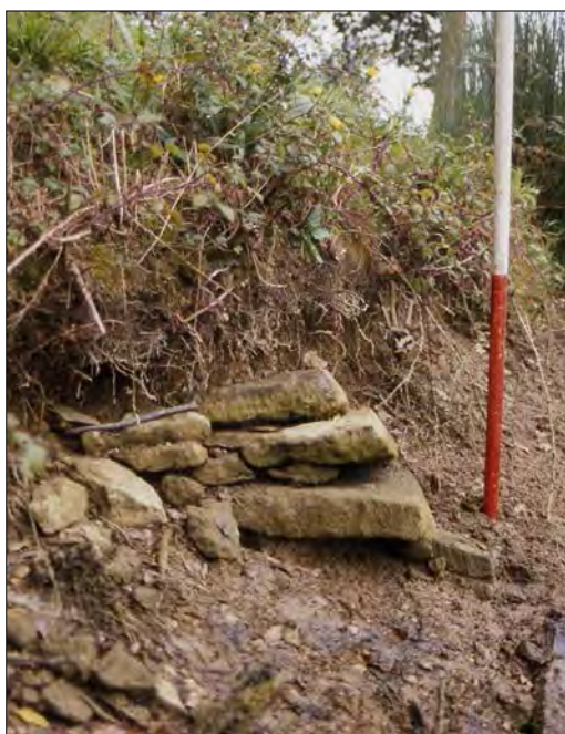
Fig.4/67 Remnants of a limestone abutment, just below SW corner of E pyramidal mount. Photograph, Brian Dix, 2000.
