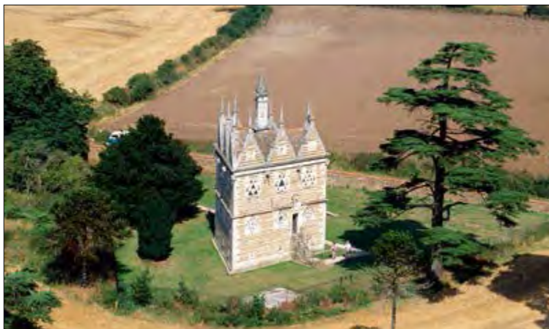
Fig.4/21 Aerial shot of the Triangular Lodge, showing the complex roof structure and dramatic skyline, filled with gables and soaring chimney
