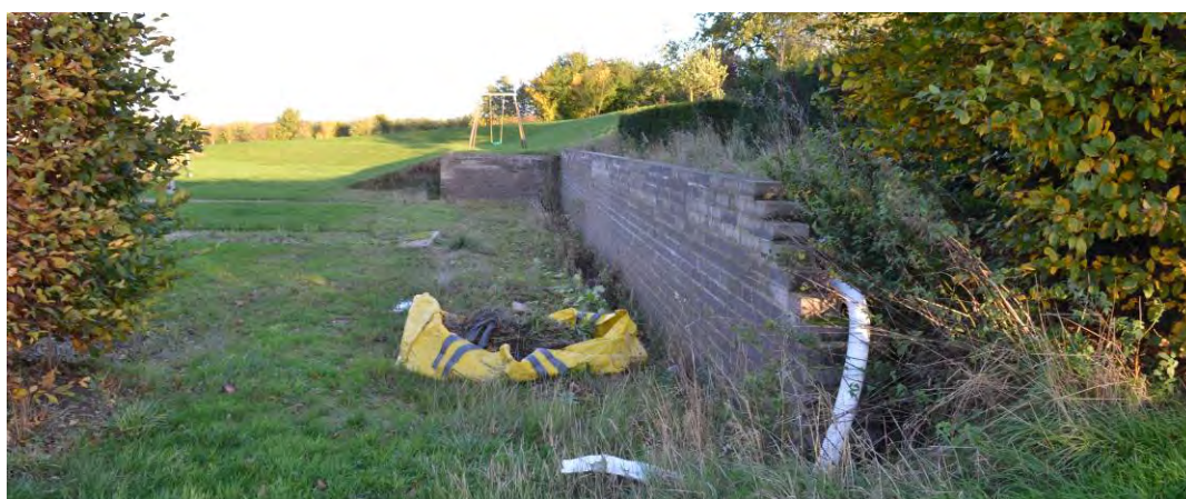
Fig. 5/25 Brick retaining wall between formal garden and tennis court (to the right), 2013
