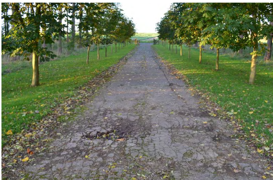
Fig.5/8 Entrance drive to Lyveden Manor, looking towards Harley Way, 2013
