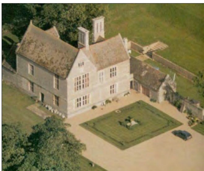
Fig.4/57 Aerial photograph of Lyveden Manor, pre-1991, showing evidence of (modified) 4 th terrace in gardens to SE of house (top right of picture)?
