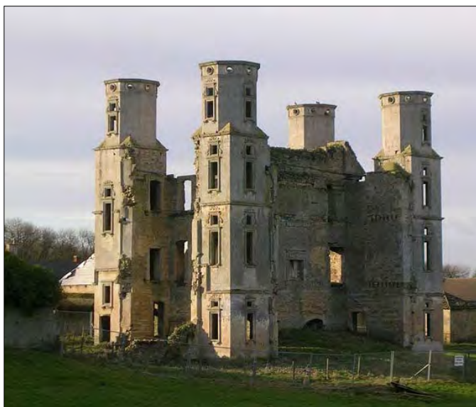
Fig.4/34 Wothorpe which Lord Exeter built in early 17 th C a mile or so from Burghley, designed on a Greek cross plan with 4 slender towers in 4 internal angles.
