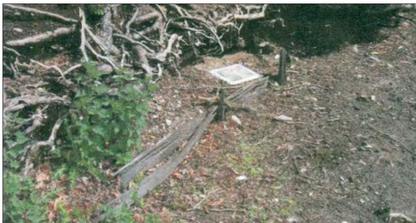
Fig.4/63 Bramshill, Hampshire, 2005, evidence of construction, with revetment, of island in lake, early 1600s (following drain-down of lake; A4 sheet of paper included, for scale).
