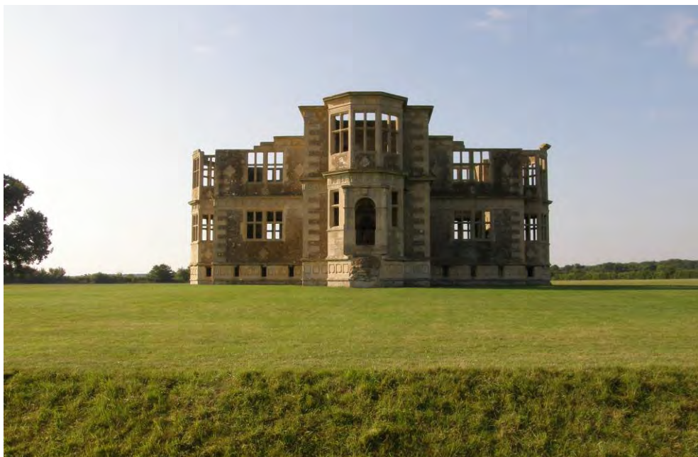
Fig.5/41 New Bield from the north, 2013
