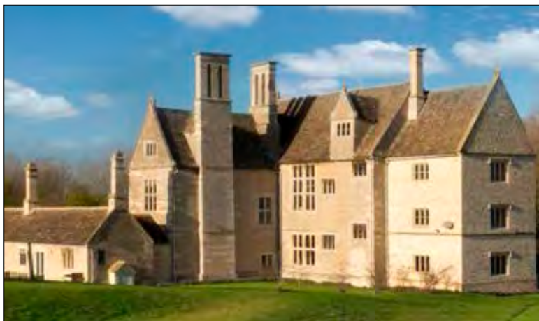
Fig.4/27 View of Lyveden Manor from the SE, showing narrow, ground floor window, tucked into the corner; evidence indicates that this was originally a doorway.
