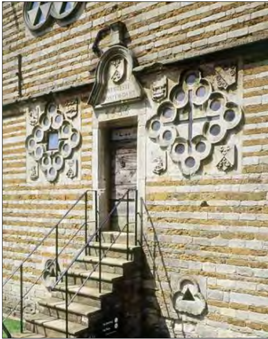
Fig.4/20 Lower storey of Tresham's Triangular (Warrener's) Lodge, Rushton, built 1594-1597, showing low trefoil windows, 'sett up' by the end of August, 1594, when the 'crosse windowes' were begun.
